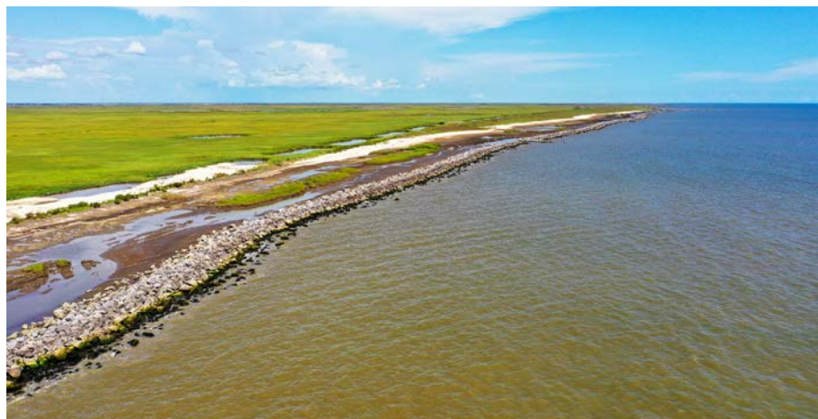
Breakwaters along the Rockefeller Shoreline
