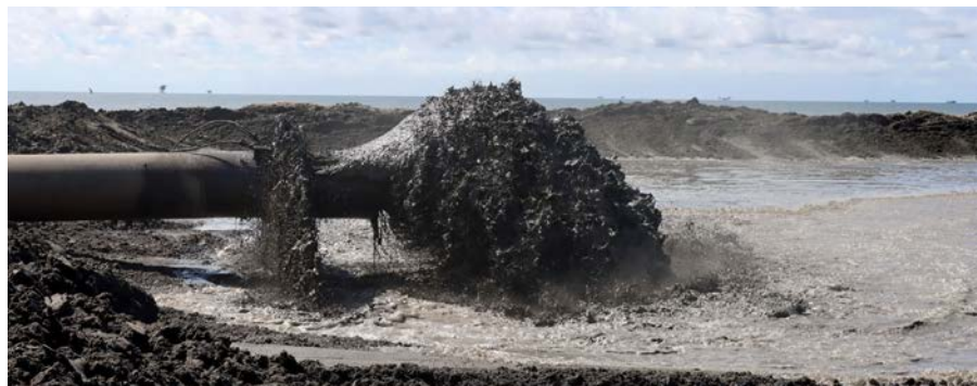
Dredge pipes pump material from the Gulf of America to Grand Isle beach
