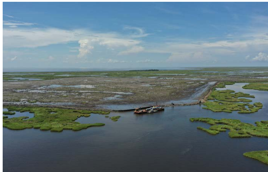
Containment cell being filled near Lake Borgne
