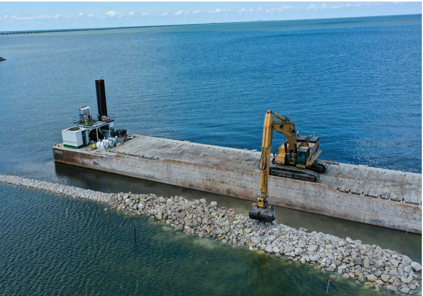
Bucktown Living Shoreline Construction
