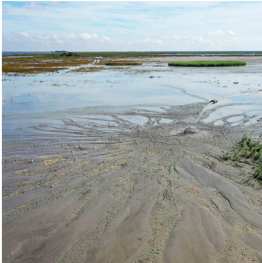
Dredging activity at Lake Borgne
