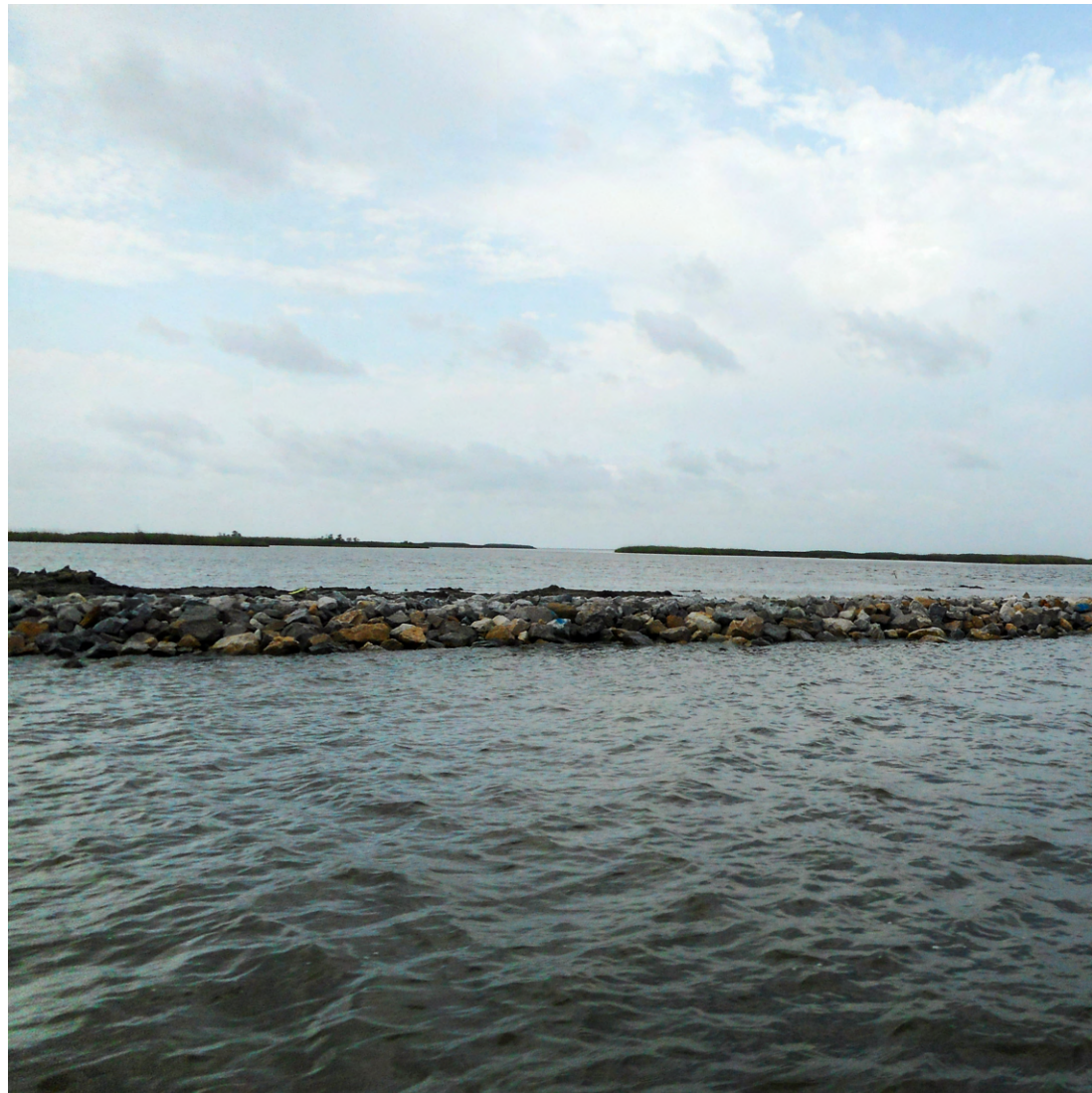
Freshwater Bayou Shoreline Protection project upon completion
