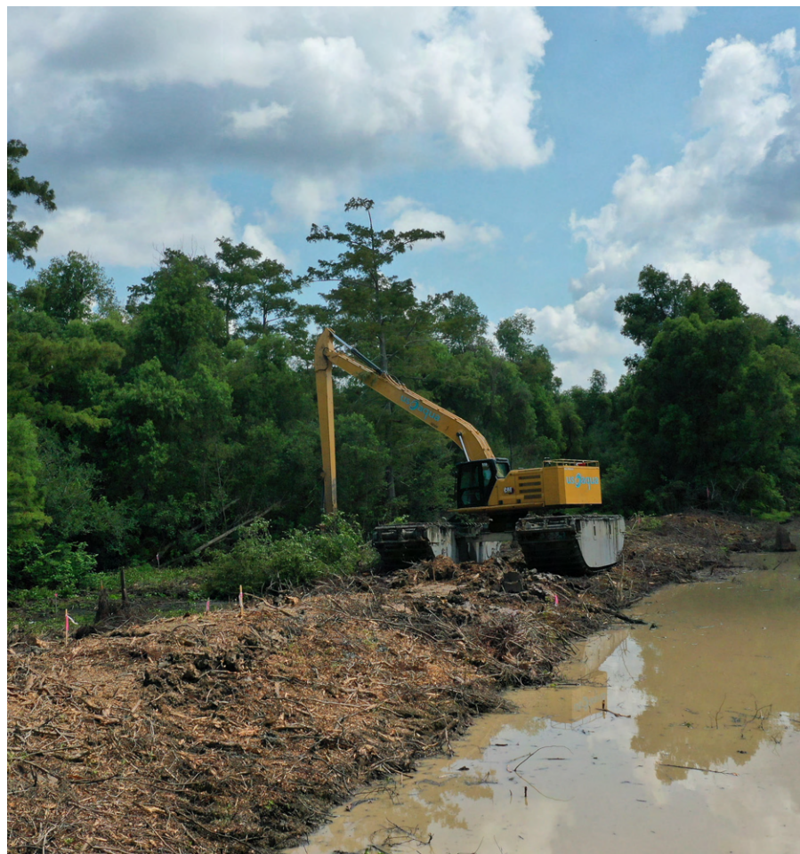
Construction of spoil bank gaps along the Dixie Corridor
