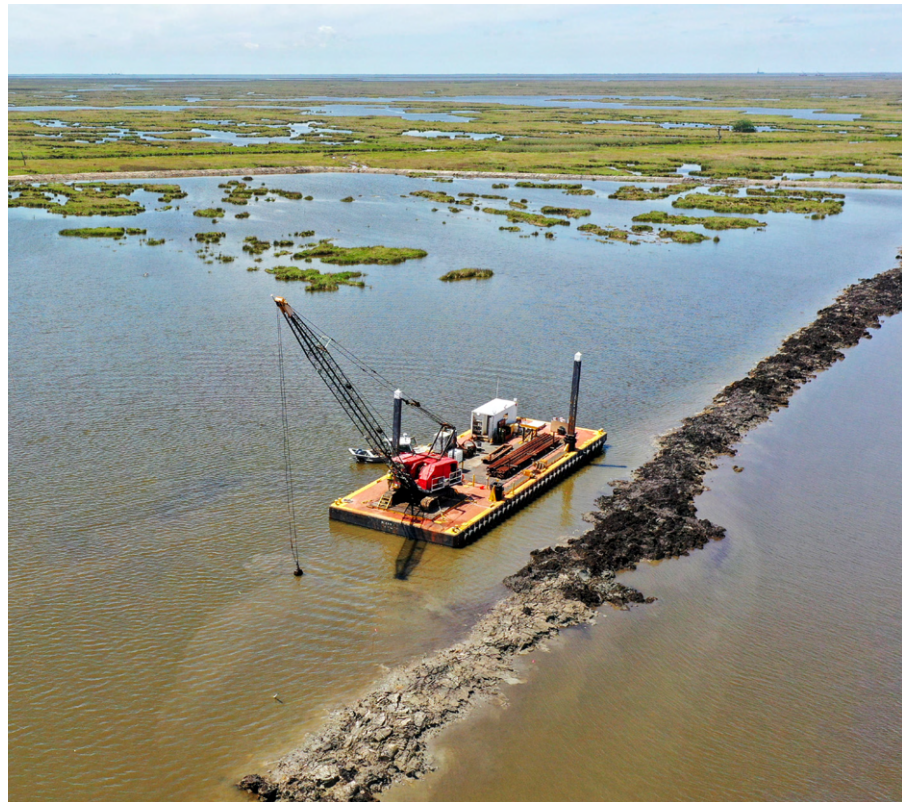
Containment dike construction at Bayou Grande Cheniere
