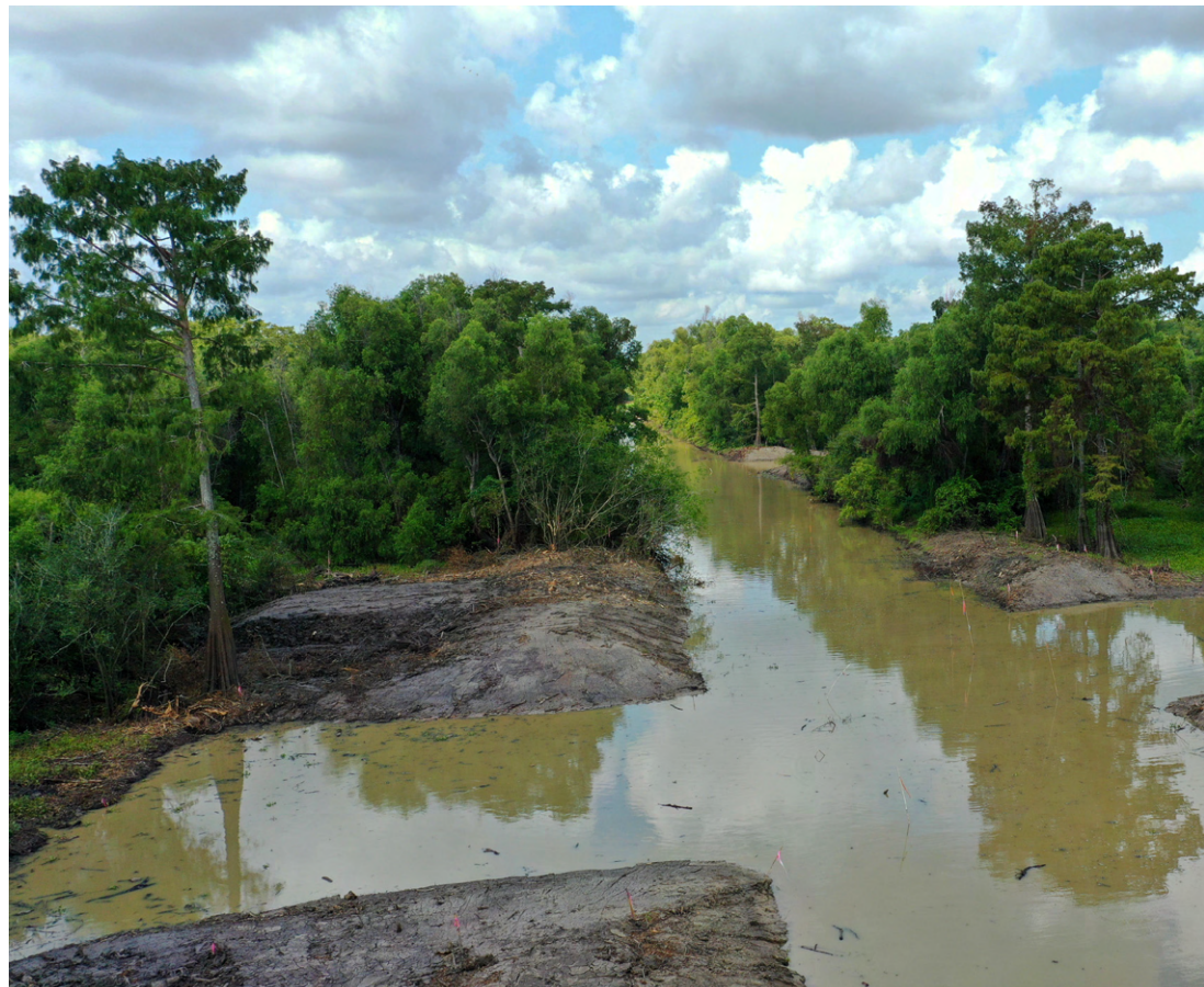
Completed spoil bank gaps along Henderson Lake's Dixie Pipeline Corridor
