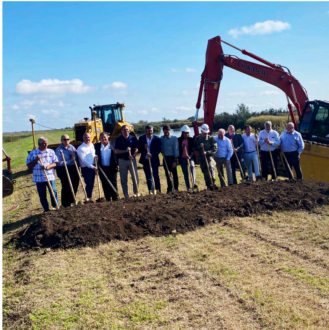
Humble Canal Floodgate groundbreaking ceremony (December 2022)
