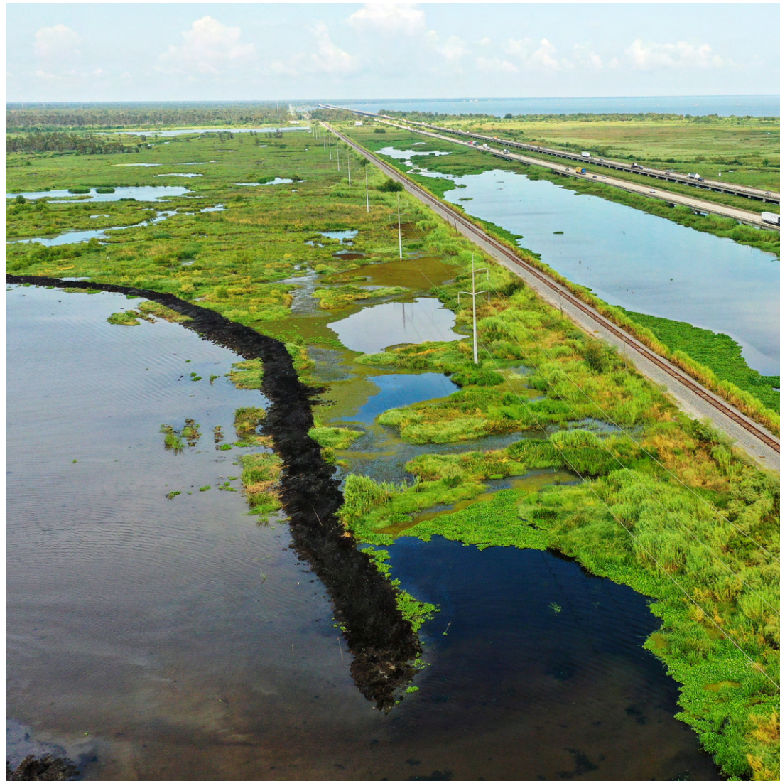
Containment dikes being constructed in the LaBranche Marsh near Interstate 10
